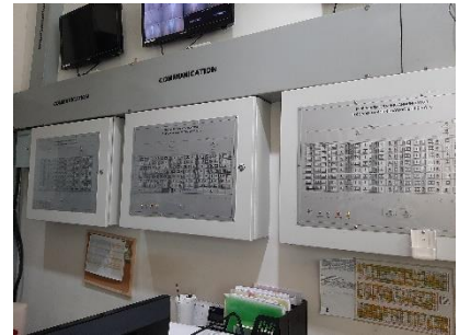
Graphic Annunciator Fire Alarm System
