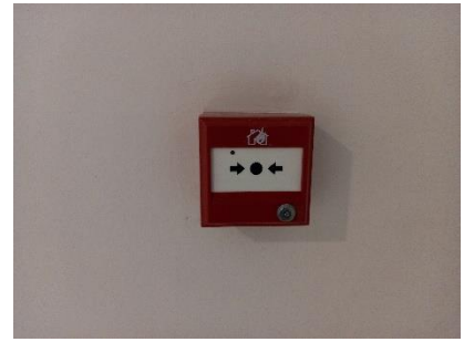
Fire Alarm Manual Station
